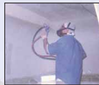
Marine adhesives being applied for wall coverings.
